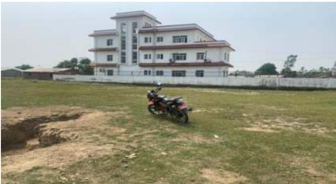
Photo 8: DHM, Kohalpur Office Building adjacent to Kohalpur Data Centre
