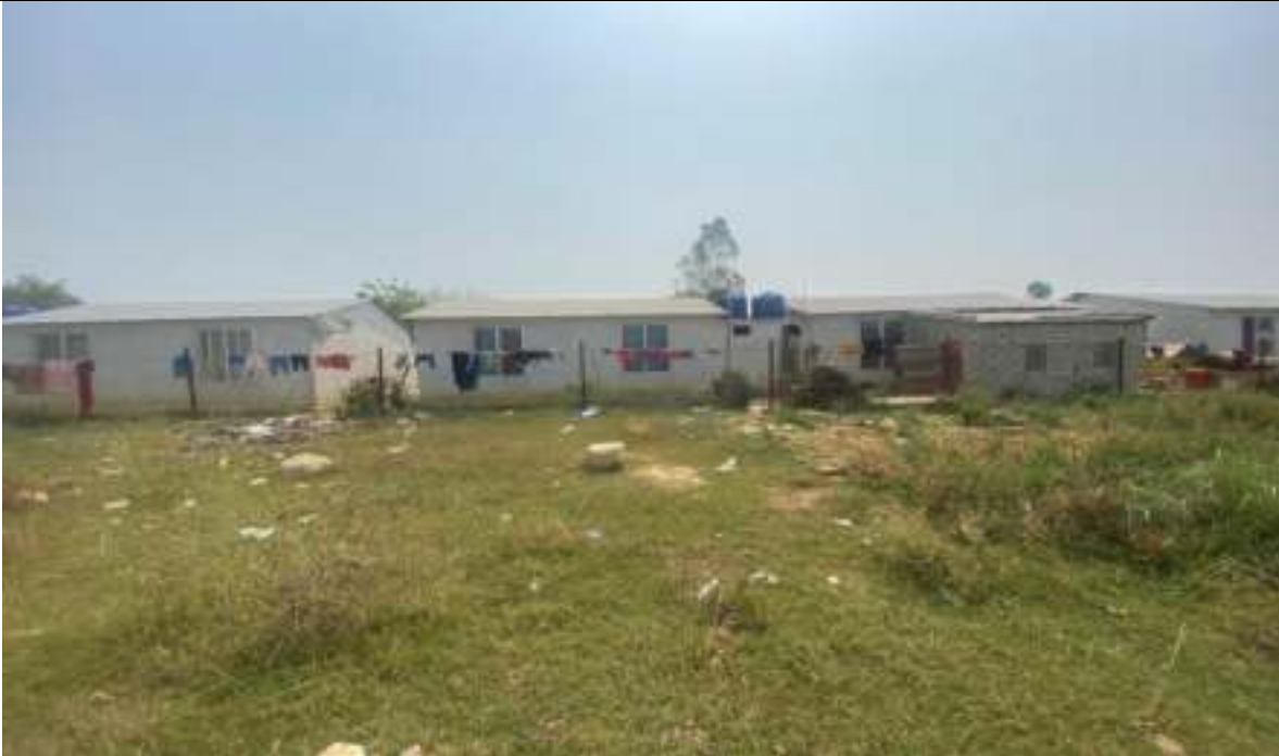
Photo 2: Kohalpur data centre location with access road
